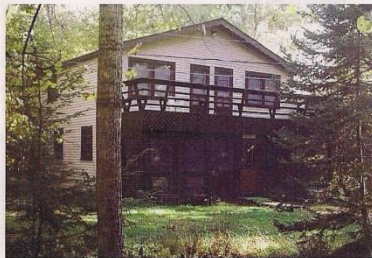
Eat-in Kitchens Large Screened-in Porches
